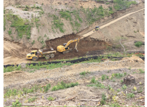
Pier 4 excavation - bridge over Curry Hollow.
