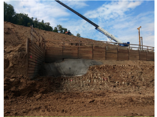
Pier 3 temporary support of excavation - bridge over Curry Hollow.
