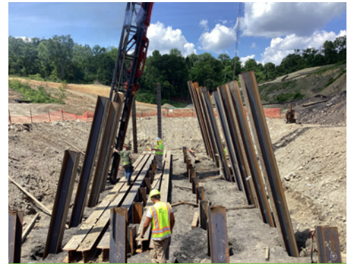
Pier 1 H-Pile driving - ramp bridge new highway to Pitt McKeesport Boulevard.
