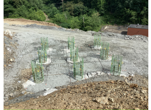
Pier 2 Caissons - bridges over Curry Hollow.
