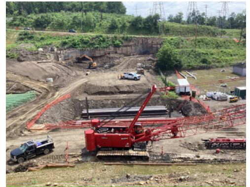
Ramp bridge new highway to Pitt McKeesport Boulevard - construction progress.
