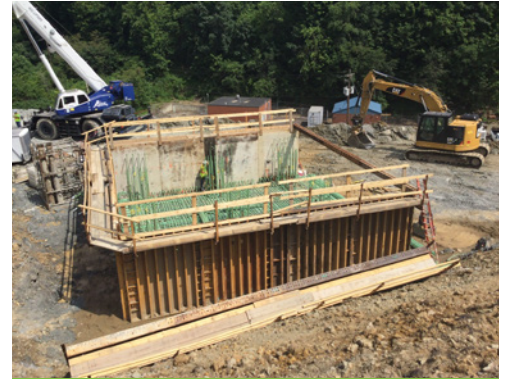
Pier 2 footing construction - bridges over Curry Hollow.
