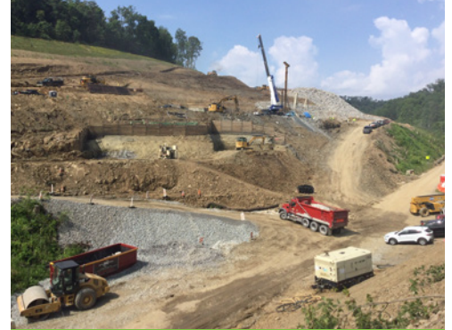
Grading Area 1 - construction activities.
