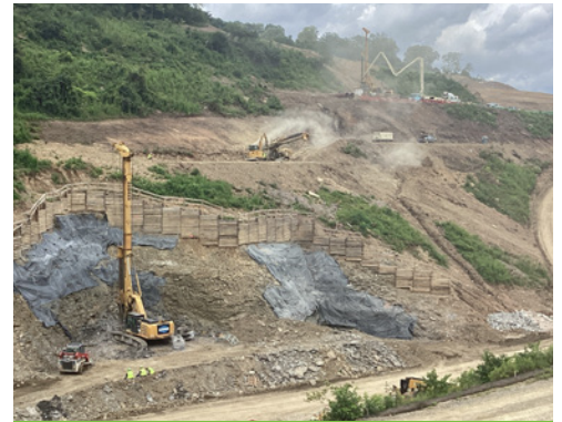
Bridges over Curry Hollow Road - Construction Progress.
