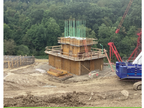
Bridges over Curry Hollow Road - MF-411B Pier 1 construction.
