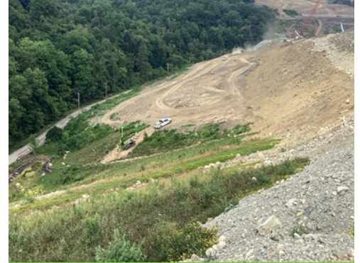
Geotechnical drilling near Camp Hollow interchange.
