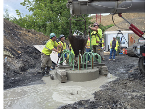
Abutment 2 H-Pile construction - ramp bridge new highway to Pitt McKeesport Boulevard.
