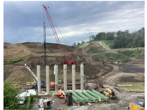
Interchange connector bridge - construction progress.
