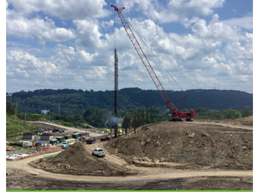
Steel H-Pile driving - interchange connector bridge.
