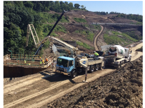
Pier 1 concrete footing placement - bridges over Curry Hollow.
