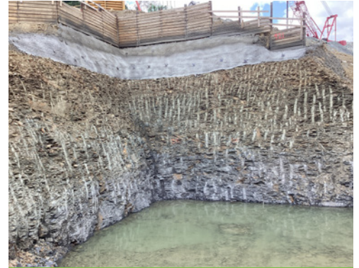
Pier 3 temporary support of excavation - bridges over Curry Hollow Road.
