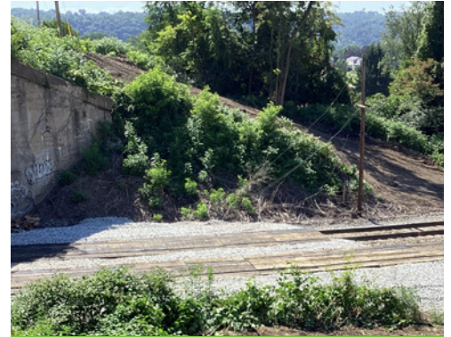
Temporary railroad crossing at Pitt McKeesport Bridge.
