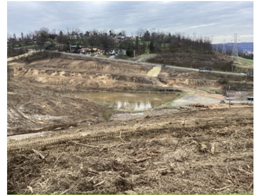
Clearing operation near Pitt McKeesport Boulevard.
