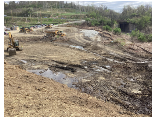
Excavation of toe bench for future embankment.
