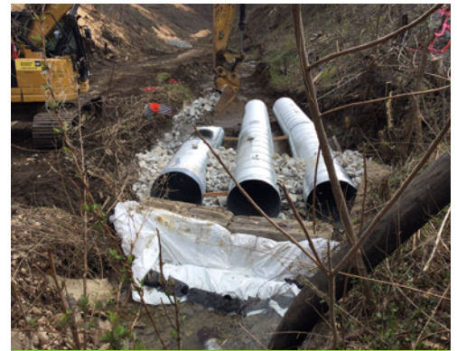
Temporary stream crossing installation.
