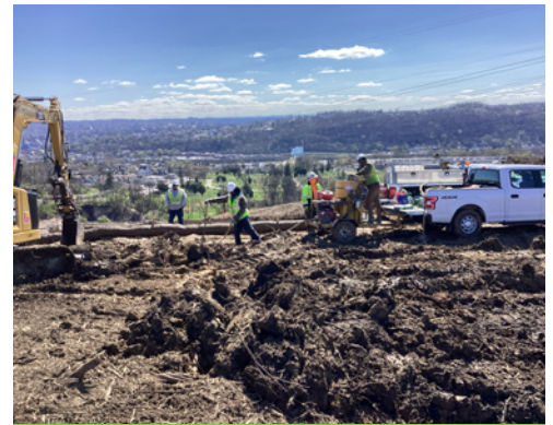
Grouting piezometer wells.
