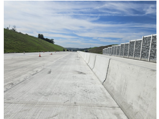
New highway looking south from Camp Hollow Road.
