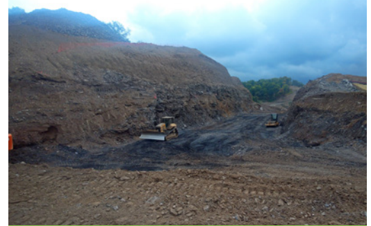
Excavation occurring between Camp Hollow Road and New England Road.
