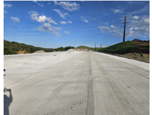
New highway looking north over Camp Hollow Road bridges.
