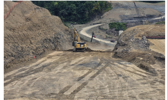
Construction progress for bridges over New England Road.
