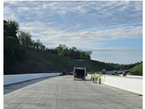
Bridges over New England Road - barrier coating.
