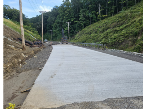
Lower Camp Hollow Road reconstruction under bridge.
