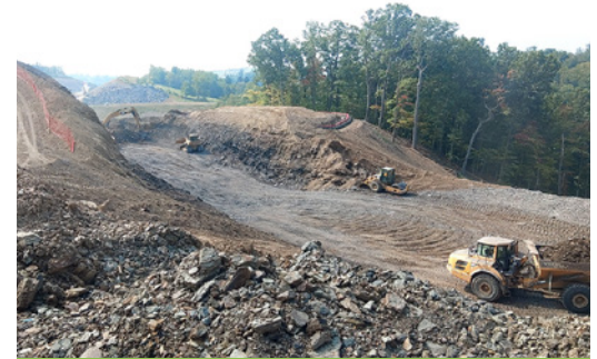
Excavation between New England Road and Camp Hollow Road.
