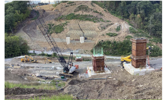
Bridges over New England Road construction progress.
