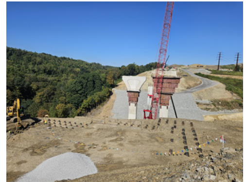
Bridges over Camp Hollow Road construction progress.
