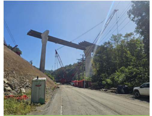
Steel girder installation for bridges over New England.
