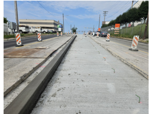
Lebanon Church Road construction progress.
