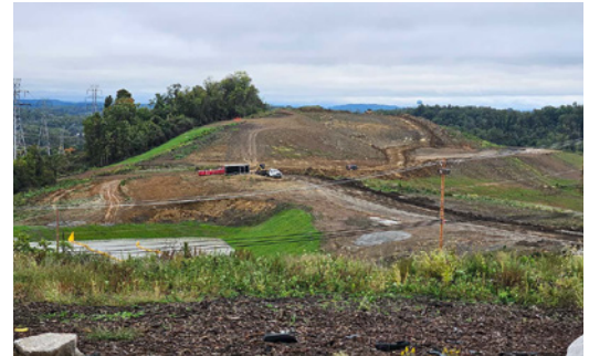
Grading Area 3 Construction Progress Near Future Camp Hollow Interchange.
