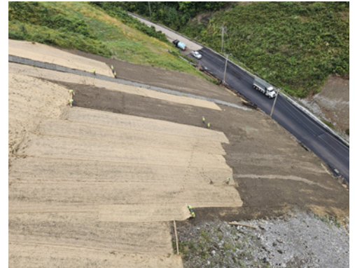
Bridges over Camp Hollow Road - straw mat installation on slope.
