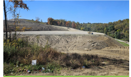
Excavation for future highway near Curry Hollow Road.
