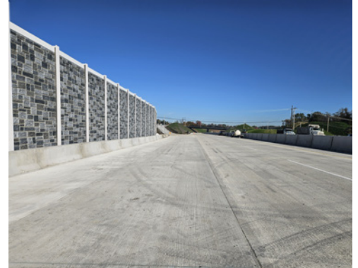
New southbound highway looking north to Camp Hollow Road interchange bridge.
