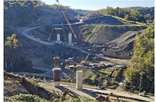
Construction progress for bridges over New England Road.
