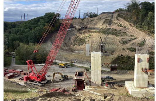
Bridges over New England Road construction progress.
