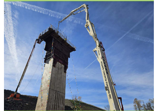
Pier 2 cap concrete placement for bridge over New England Road.
