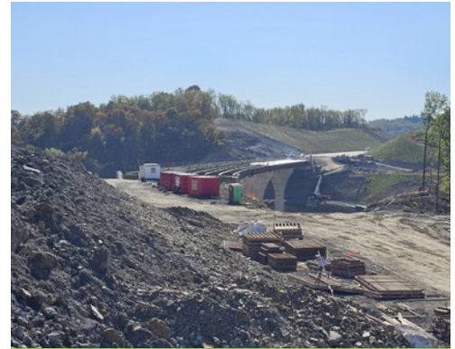
Bridges over New England Road - construction progress.
