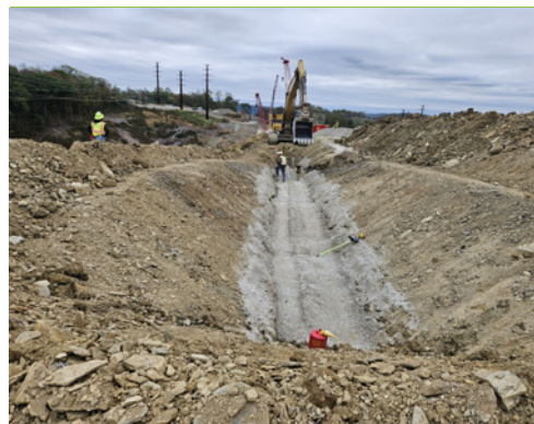
Stormwater drainage pipe installation.
