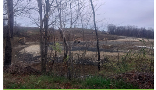
Embankment construction near Curry Hollow Road.
