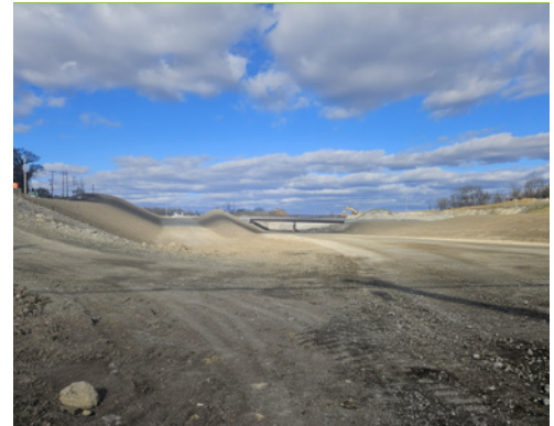
Future mainline alignment under Camp Hollow Road.
