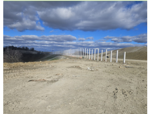
Sound wall construction along new alignment.
