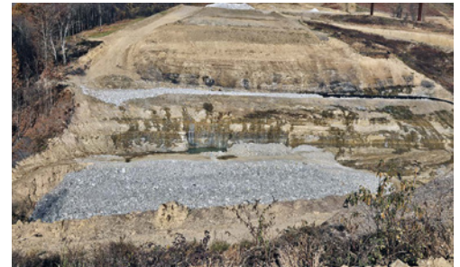
Slope excavation for future bridges over Camp Hollow Road.
