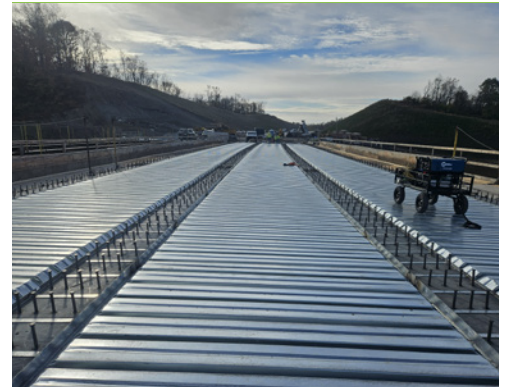
Bridges over New England Road - bridge deck form installation.
