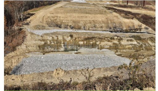
Future location of bridges over Camp Hollow Road.
