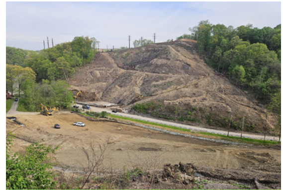
Bridges over New England Road construction progress.
