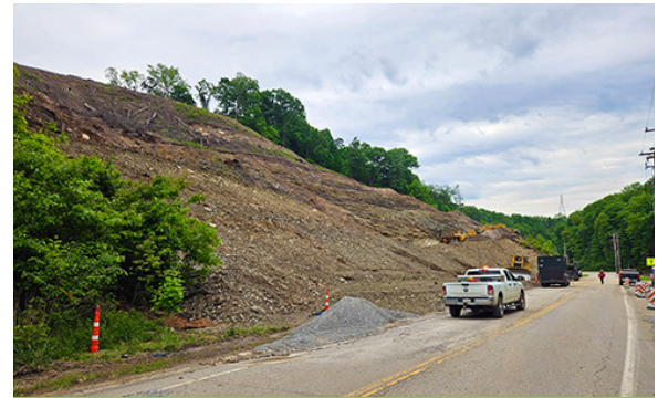
North slope MF-406-407 (bridges over New England Road).
