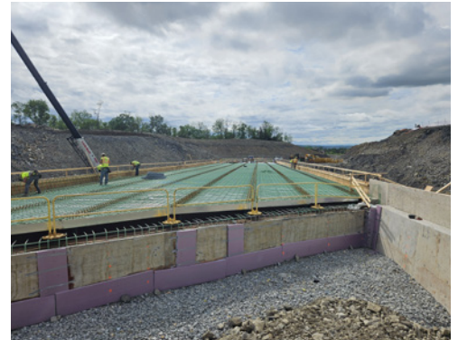
Preparation for concrete bridge deck placement future Camp Hollow Road bridge.
