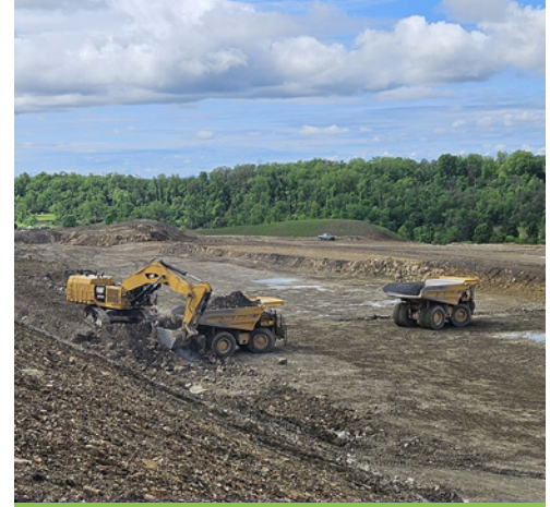
Excavation for new highway alignment.
