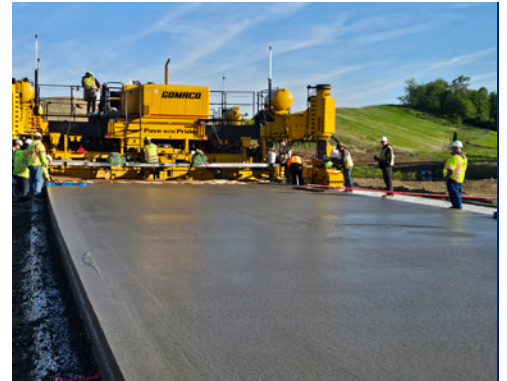
New highway concrete paving.
