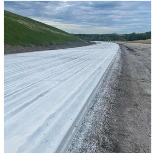
New highway concrete pavement.
