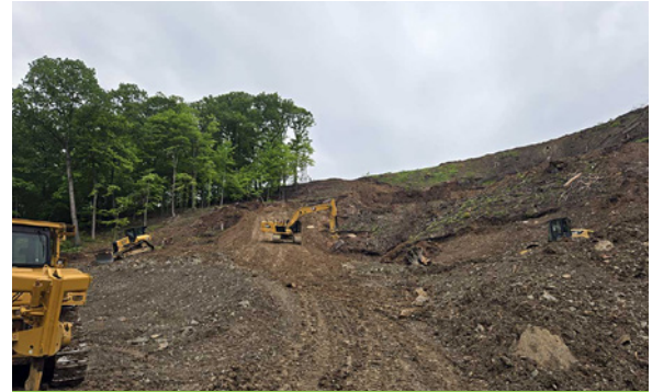
Excavation north of New England Road.
