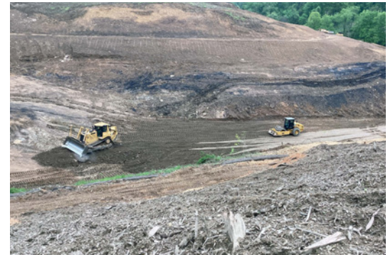
Excavation beginning for future sediment basin.
