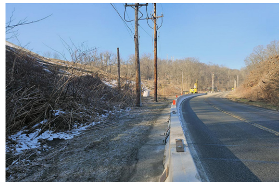
New England Road maintenance and protection of traffic.
