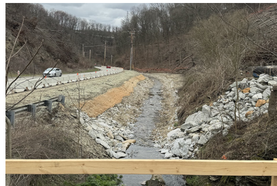
MON 2-S24 stream relocation along New England Road complete.
