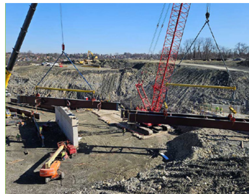
Steel girder erection for future Camp Hollow Road bridge.
