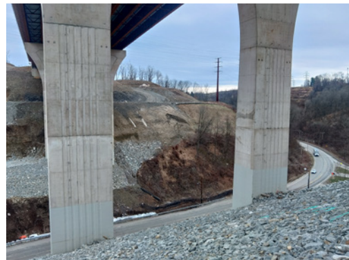
View of Camp Hollow Road under new bridges.
