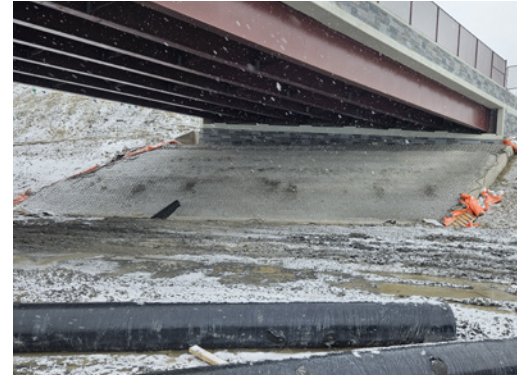
Bridge carrying Camp Hollow Road - abut 1 slope wall.
