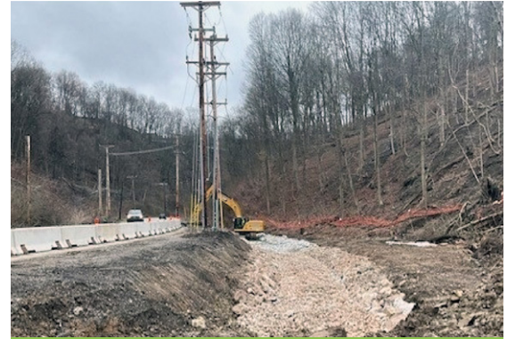
Pine Creek stream relocation adjacent to New England Road.
