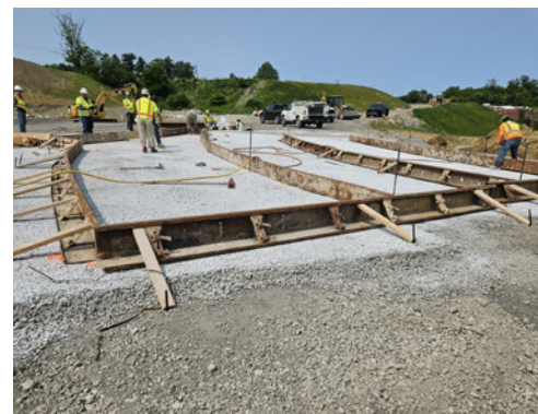
Preparing for concrete placement for Camp Hollow Road roundabout.
