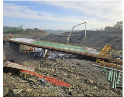
Concrete bridge deck placement - future Camp Hollow Road bridge.
