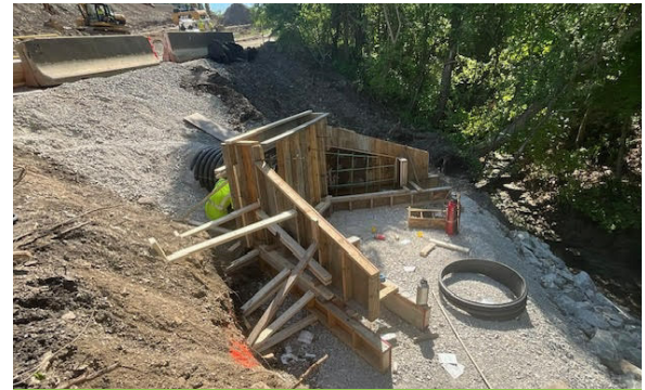
Pipe culvert endwall form work.
