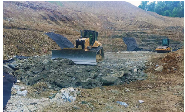
Placing fill for New England Road bridges.
